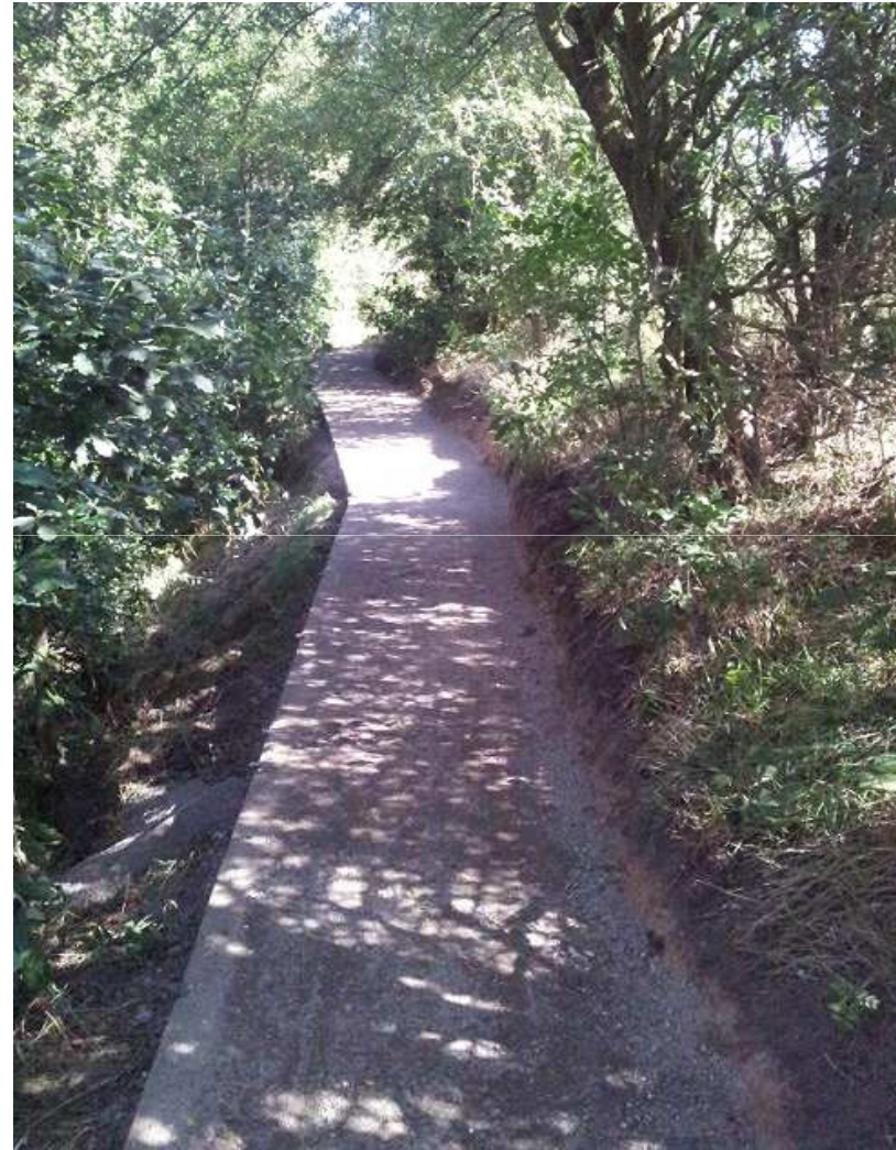
Path construction – Rawmarsh
